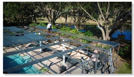
Clean the frame: Once the old screen is removed, the frame should be thoroughly cleaned to remove any dirt, debris, or old spline that may be stuck to it. This is done with a pressure washer and elbow grease. This is not a step done casually or quickly: see
